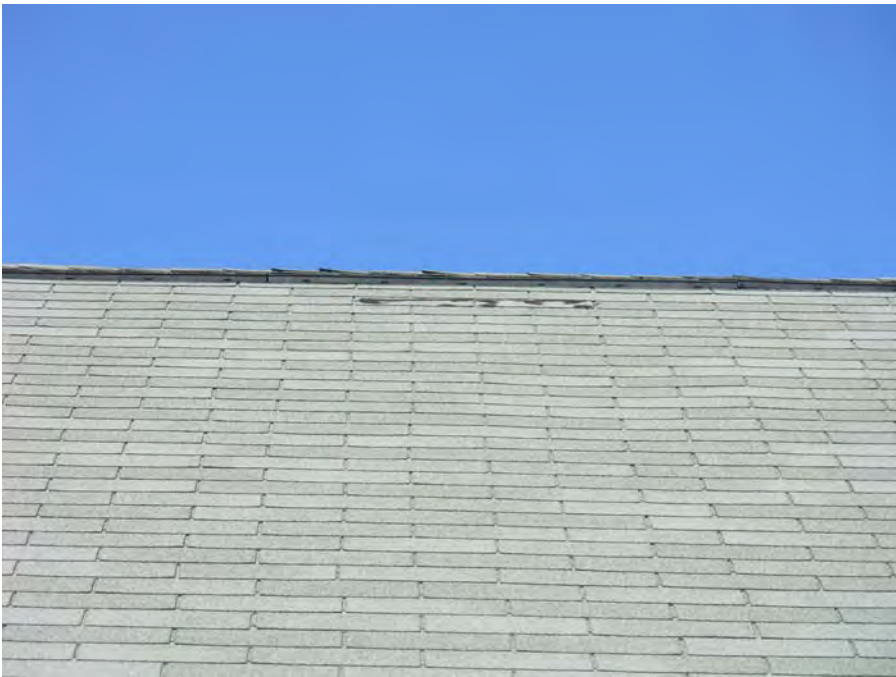
5. Spot missing and lifting roofing shingles
