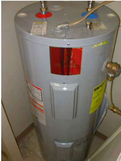
15. Typical unit DHW tanks
