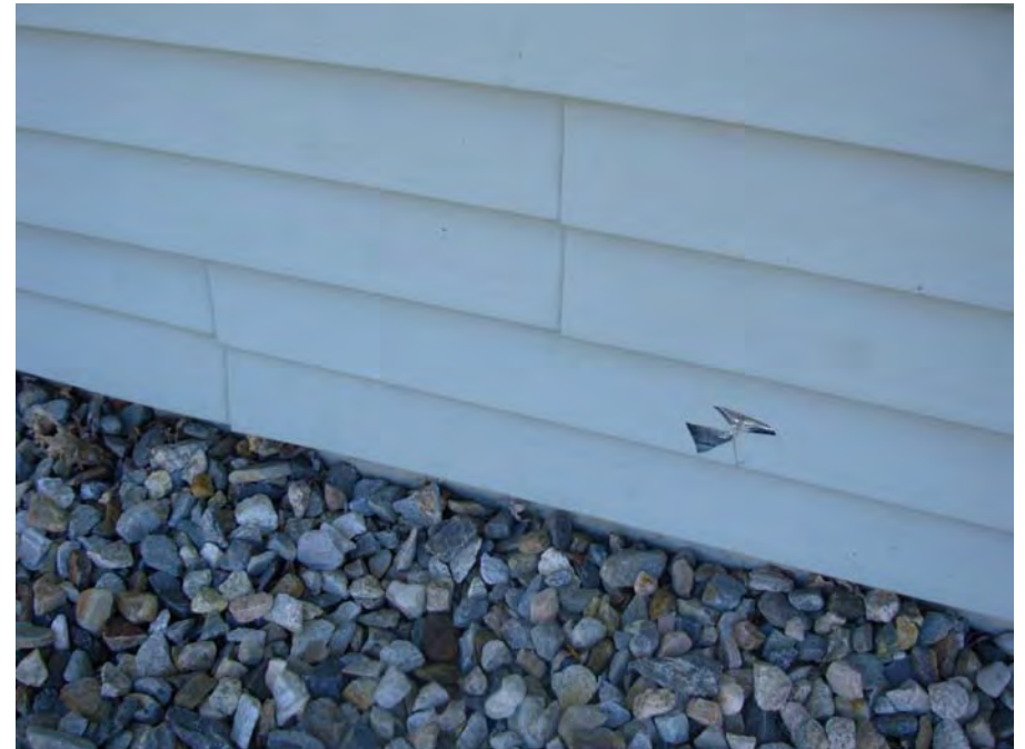
4. Minimal vinyl siding damage
