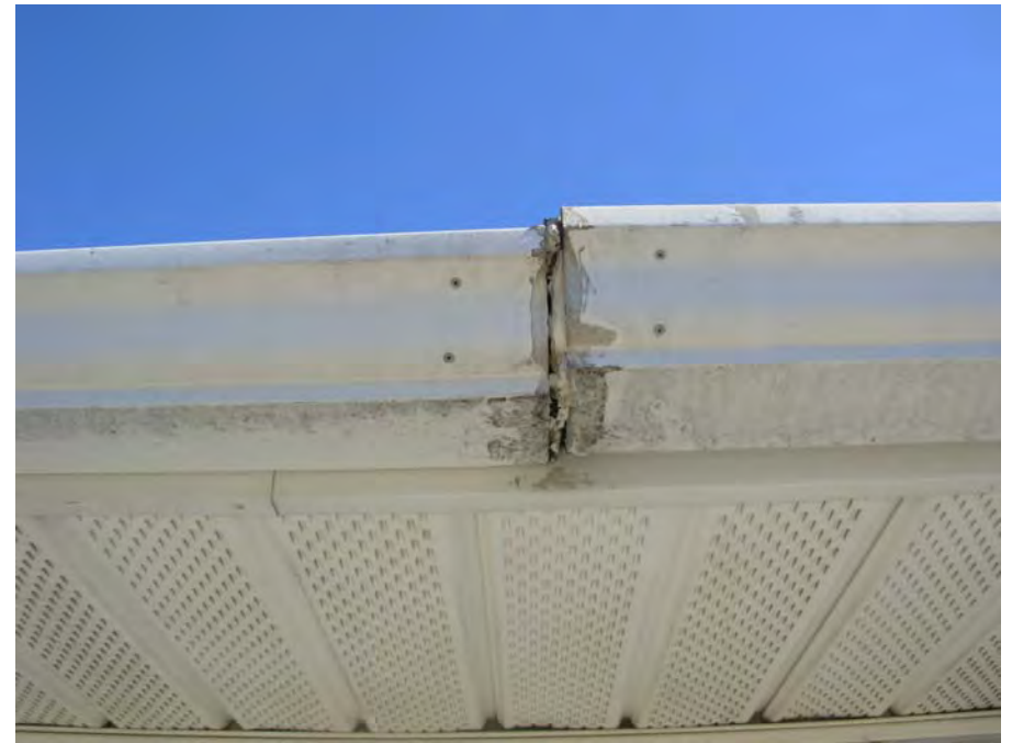
6. Gutter seams separating at several locations
