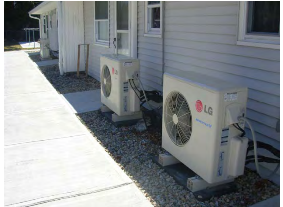
16. Heat pump HVAC system exterior condensers, typical
